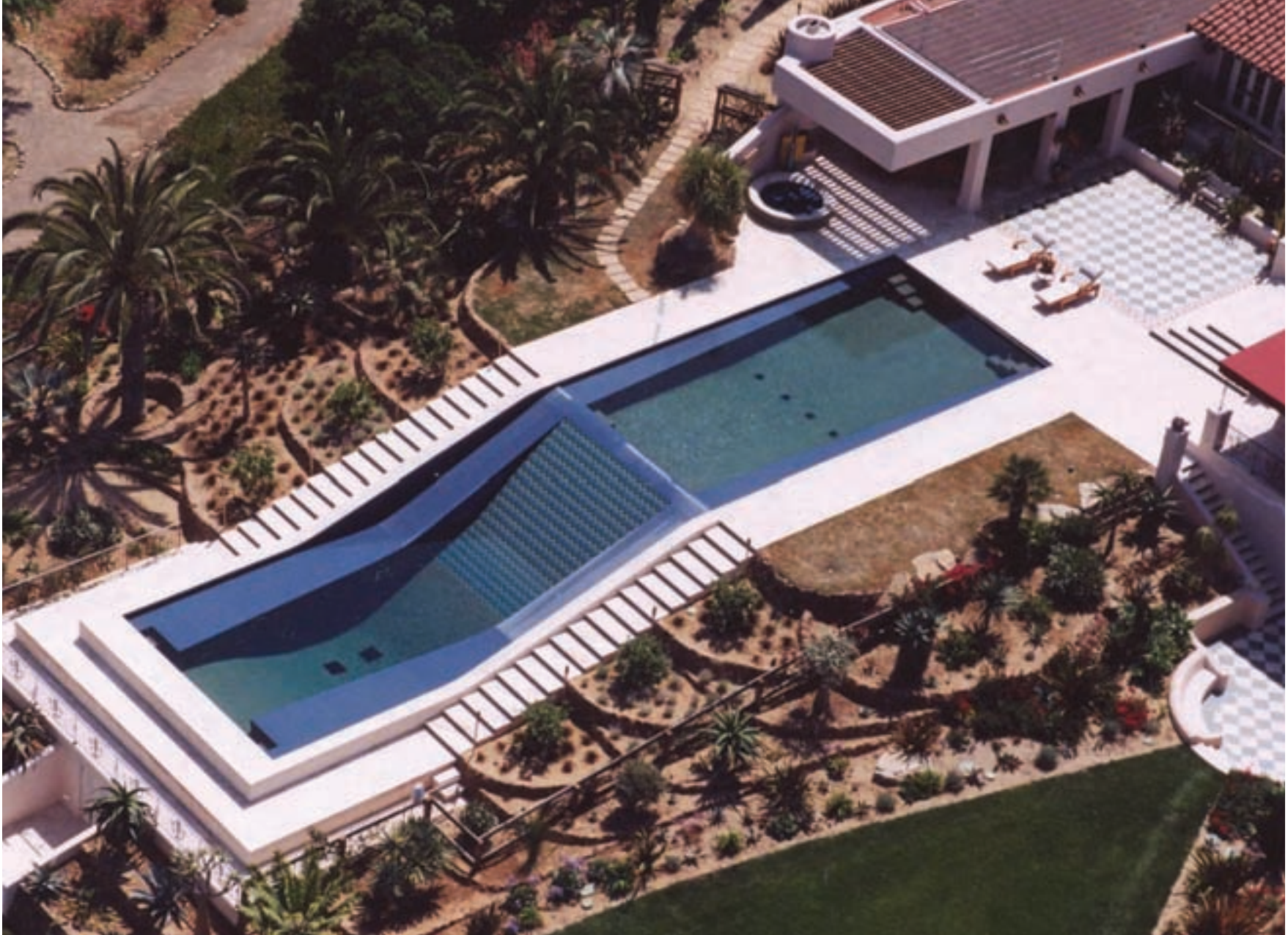
Exceptional in its design, this pool is 85-feet in length and features a large upper play pool with a 22-foot negative edge and a 10-foot deep diving pool below. Twin 7 hp pumps send 600 gpm over the tiled mosaic slide, allowing users to literally swim over the negative edge and into the 10-foot deep pool below. Both pools are protected by a single giant motorized safety cover. Photo courtesy of Mission Pools, Escondido, California
