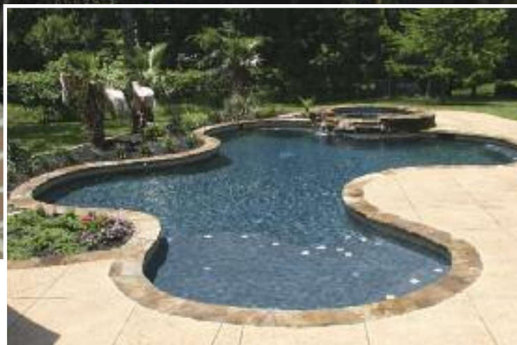
Stamp overlay decking and chocolate flagstone coping surround this freeform pool, which has a dark navy exposed aggregate interior. Natural boulders form the spa's spillway, and white tiles accent the Baja shelf and underwater benches.
