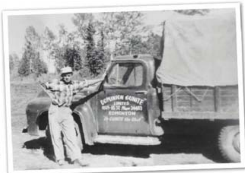
When the company was originally founded in 1955, it specialized in shotcrete (gunite) for tunnels and retaining walls.
